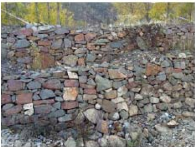
渣场生态恢复挡墙
